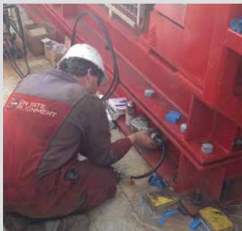
We perform controlled tightening of bolted connections, calculating the torque according to industry best practices and classification rules.
